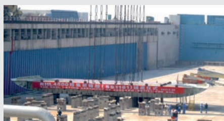
Keel-laying of the first double bottom
